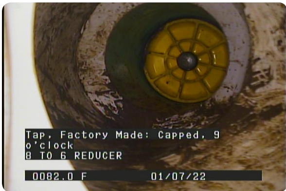
Tap, Factory Made: Capped at 082.0 feet, 9 o'clock, 6 in | 8 TO 6 REDUCER
