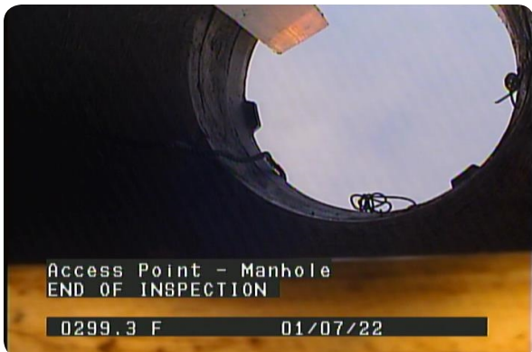
Access Point - Manhole at 299.0 feet | END OF INSPECTION
